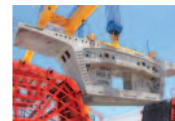
Precast pier segment being lifted in casting yard
