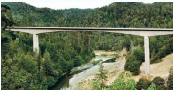
(Photo Courtesy of FINLEY Engineering Group, Inc.)
