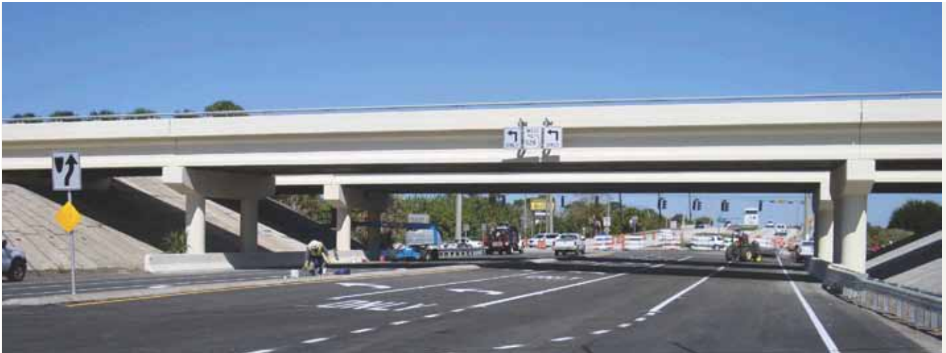
The repaired bridge was completed 3 days ahead of schedule, restoring critical access to key areas, including the Kennedy Space Center, Port Canaveral, and Cocoa Beach.
