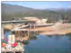
View of Lake Shasta from atop Pier 2
