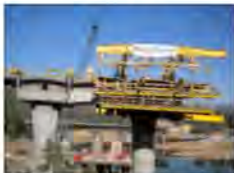
The first of 4 Form Travelers is sitting on Pier 2
