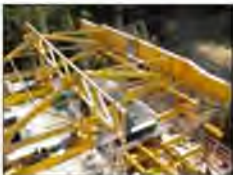
Aerial view of the form travelers at Pier 2
