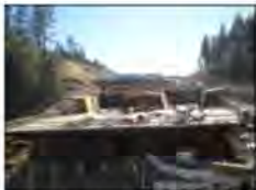
End Span Falsework and segment forms
