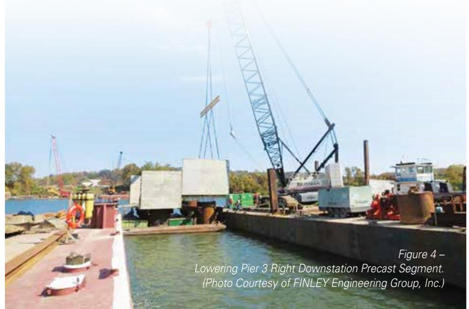
Figure 4 – Lowering Pier 3 Right Downstation Precast Segment. (Photo Courtesy of FINLEY Engineering Group, Inc.)
