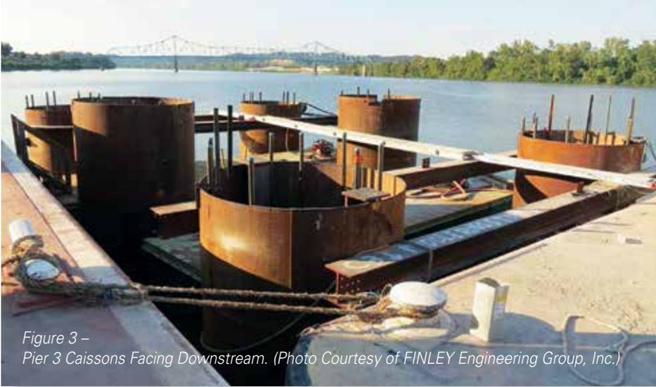
Figure 3 – Pier 3 Caissons Facing Downstream. (Photo Courtesy of FINLEY Engineering Group, Inc.)
