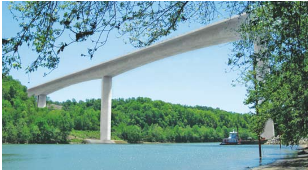
Figure 1 – The Pennsylvania Turnpike Monongahela River Bridge is being built in balanced cantilever construction to cross the river, rail lines and local roads. (Rendering Courtesy of FIGG)
