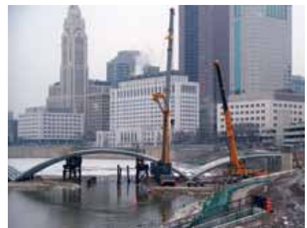
Snow flurries did not stop construction of the top segment of the rib arch on the Rich Street Bridge. Photo: Ohio Department of Transportation District 6.
