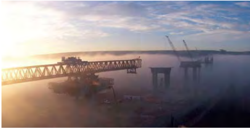
Figure 14 - Otay River Bridge (photo courtesy of International Bridge Technologies, Inc.).
