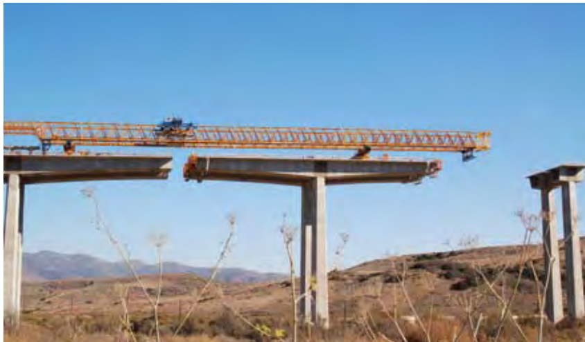
Figure 15- Otay River Bridge (photo courtesy of International Bridge Technologies, Inc.).
