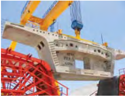
Figure 20 - Pier Diaphragm Segment Road 431 Bridge (photo courtesy of FEG).
