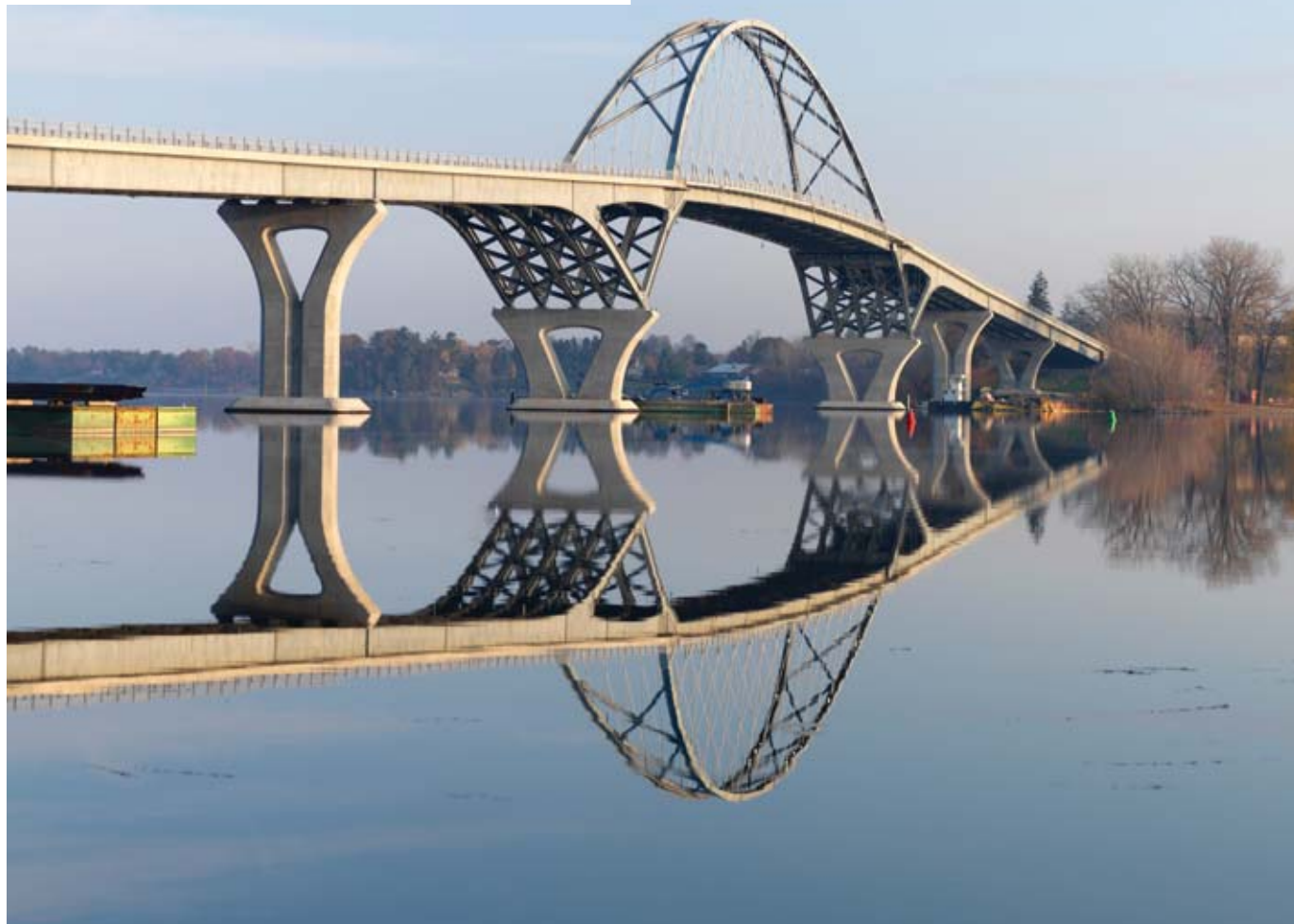
The new Lake Champlain Bridge, connecting Crown Point, N.Y., and Chimney Point, Vt., replaces the 80-year-old bridge that was found to be deficient.
