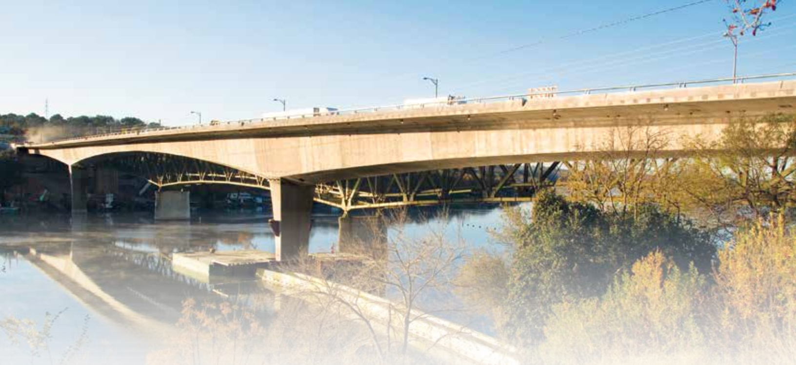
Figure 10 – US 281 Colorado River Bridge over Lake Marble Falls. (Photo Courtesy of Archer Western Contractors)
