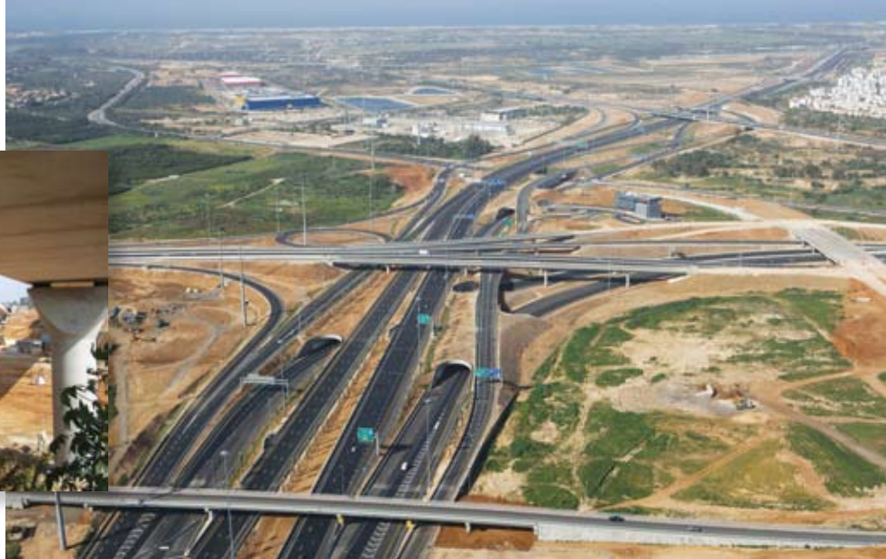
Aerial view of the Ein Ha'kore Interchange of Road 431. Precast concrete segmental bridges offer insights into how durability and sustainable construction intertwine. Photo: Danya-Cebus.
